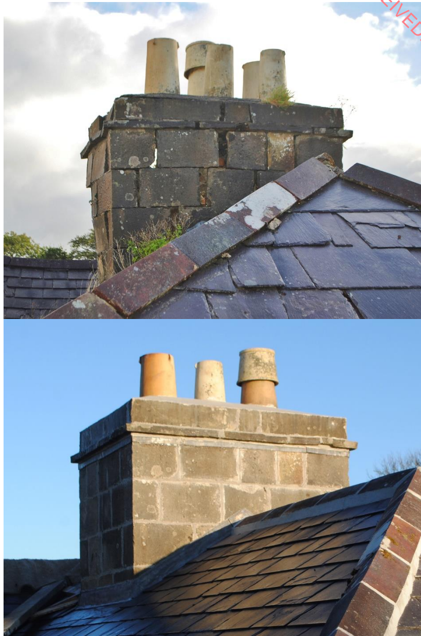
Figures 10-11: A photograph illustrating the poor condition of the central chimney stack in May 2016 with light visible through dislodged stone work. The limestone was numbered and carefully dismantled to allow for a faithful reconstruction with each stone returned to its original position and repointed using a lime mortar
