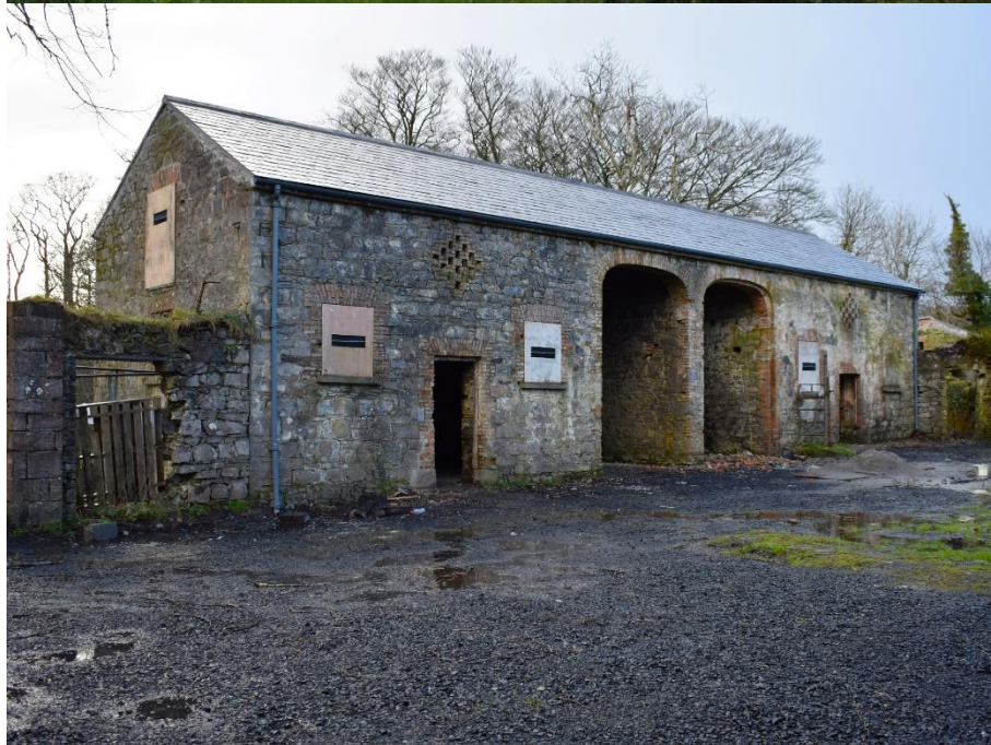
Figures 20-21: The outbuilding had fallen into ruins by 2010, its exterior covered in ivy, its interior a forest of brambles. The first phase of restoration has included the removal of vegetation, the rebedding of loose and missing masonry and the construction of a new roof with cast-iron rainwater goods
