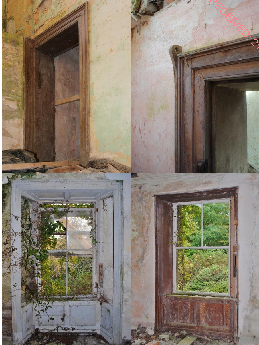
Figures 6-9: Although increasingly exposed to the elements, and subjected to theft and vandalism, the interior nevertheless retains original features of interest including, clockwise, an unusual architrave framing a corner door opening; a second architrave with integrated brackets for a draught curtain rod; an architrave around a window in the dining room with a simple moulded plasterwork cornice overhead; and an architrave with panelled reveals and shutters framing a window in one of the bedrooms on the first floor
