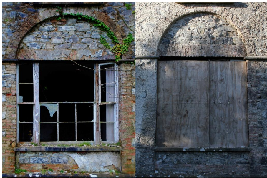
Figures 14-15: A tripartite window opening in a Morrison-esque recess originally allowed the occupants to enjoy scenic views overlooking manicured grounds. Although in poor repair, and with much of the glazing broken or missing, the hornless frames may potentially be restored or, at the very least, used as templates for period-appropriate replacements when work on the next stage of restoration takes place. In the meantime, plywood sheets, perforated to allow for ventilation, prevent unauthorised access into the glebe house and the further deterioration of its original fabric
